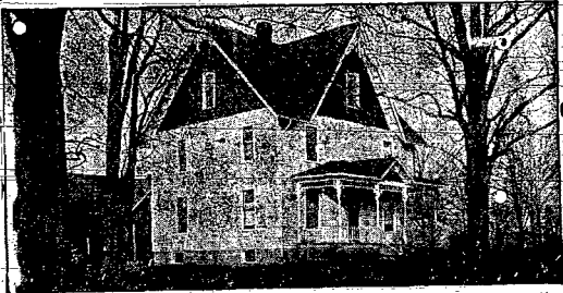
House with Furnace and Bath on Farm No. 8104. Large, new barn.
